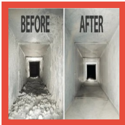
Duct Cleaning Services
