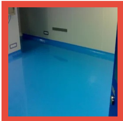
Epoxy Coving Services
